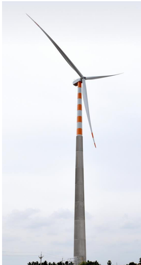
Suzlon's S120-140m WTG with 140 meters Hybrid Concrete Tubular Tower at Tirunelveli,
